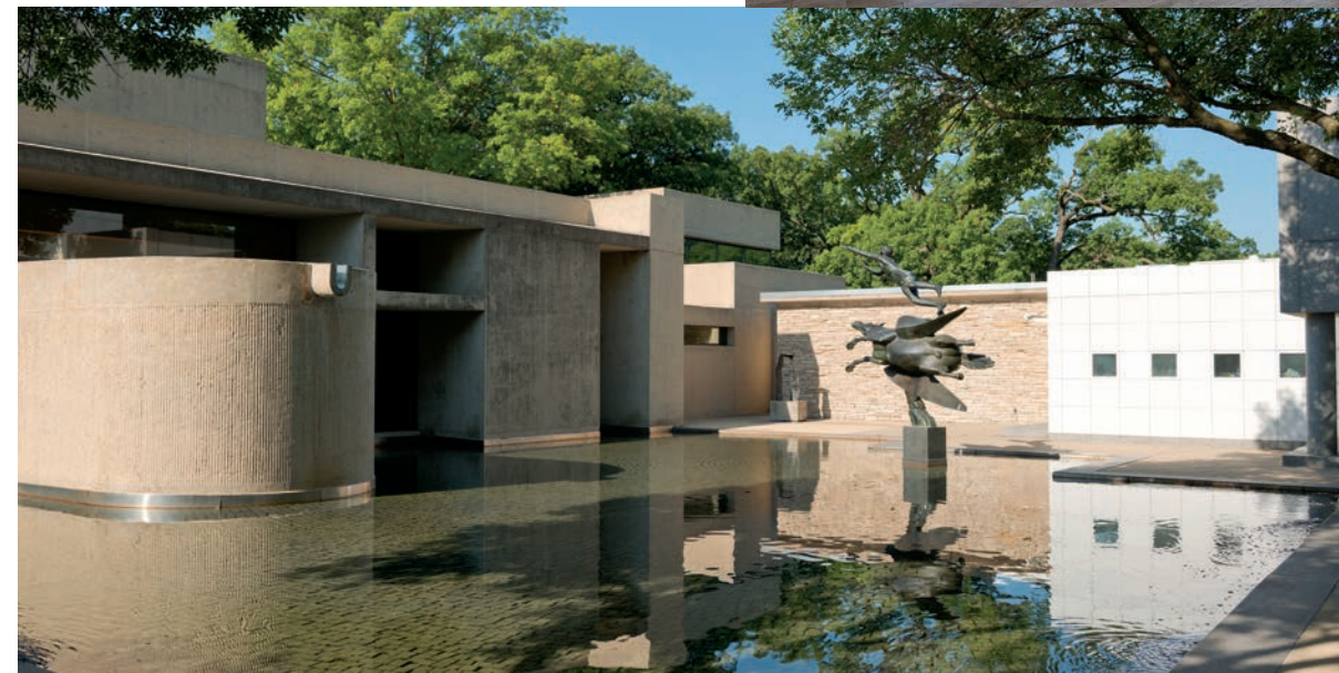
TOP The concrete "wings" of the butterfly roof overhead admit abundant natural light which cascades over the roughened concrete walls. Photo: Paul Crosby
